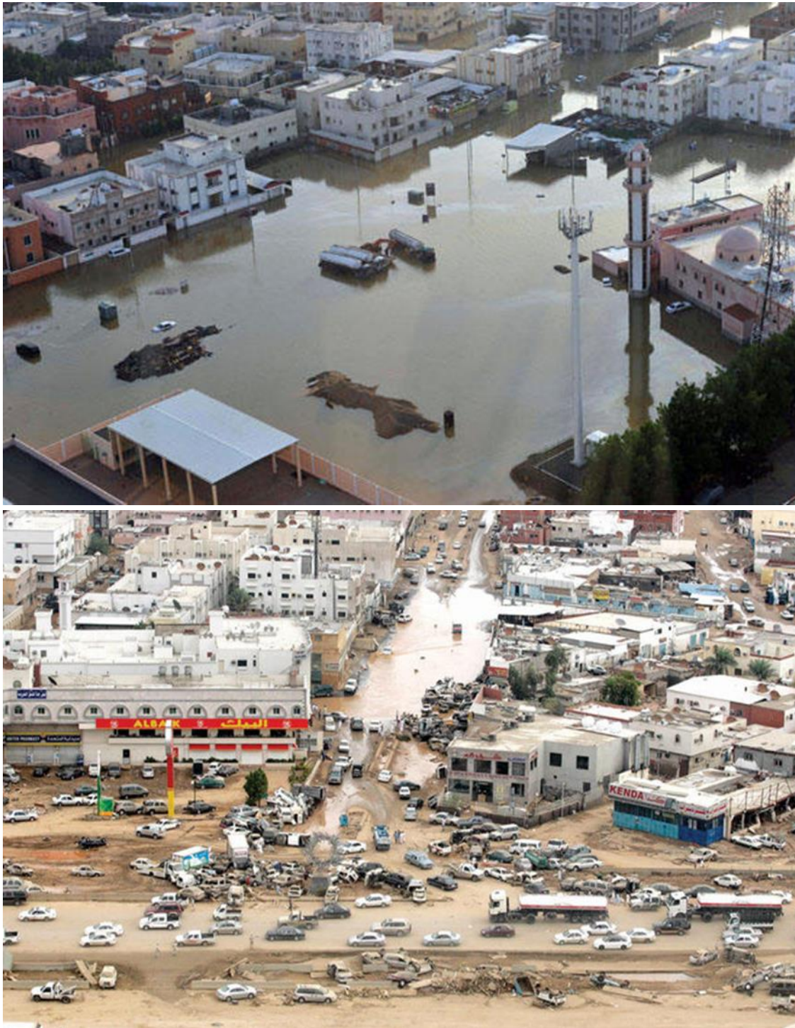
Figure. Views of Jeddah in the aftermath of 2009 floods
